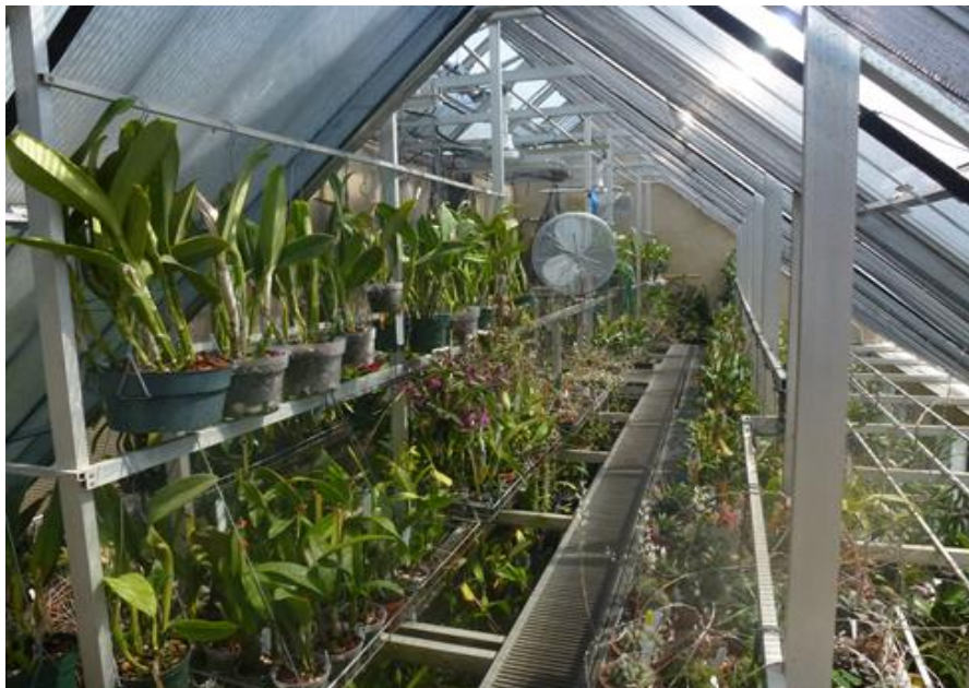
Upper floor. Also well-known as the 'BURN ZONE'. Access by circular stair. Galvanized steel walkways supported by bottom cords of custom designed aluminum spanning trusses. Plants are suspended in galvanized metal trays and are hung from two levels of aluminum cross tubes. North wall has \frac{3}{4} " expanded metal wire for hanging. Both manual and motor operated ridge vents. Two 24" oscillating fans with 6 misting nozzles each utilized for humidification, and cooling. New 65% shade cloth.
